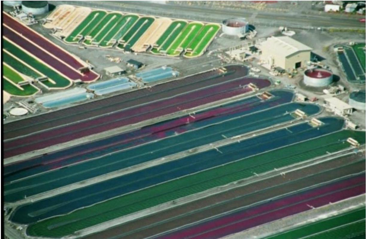
Figure 3. Cyanotech Corporation natural *Haematococcus* algae astaxanthin production facility in Kailua-Kona, Hawaii. The large ponds hold approximately 500 cubic meters of algal culture.
